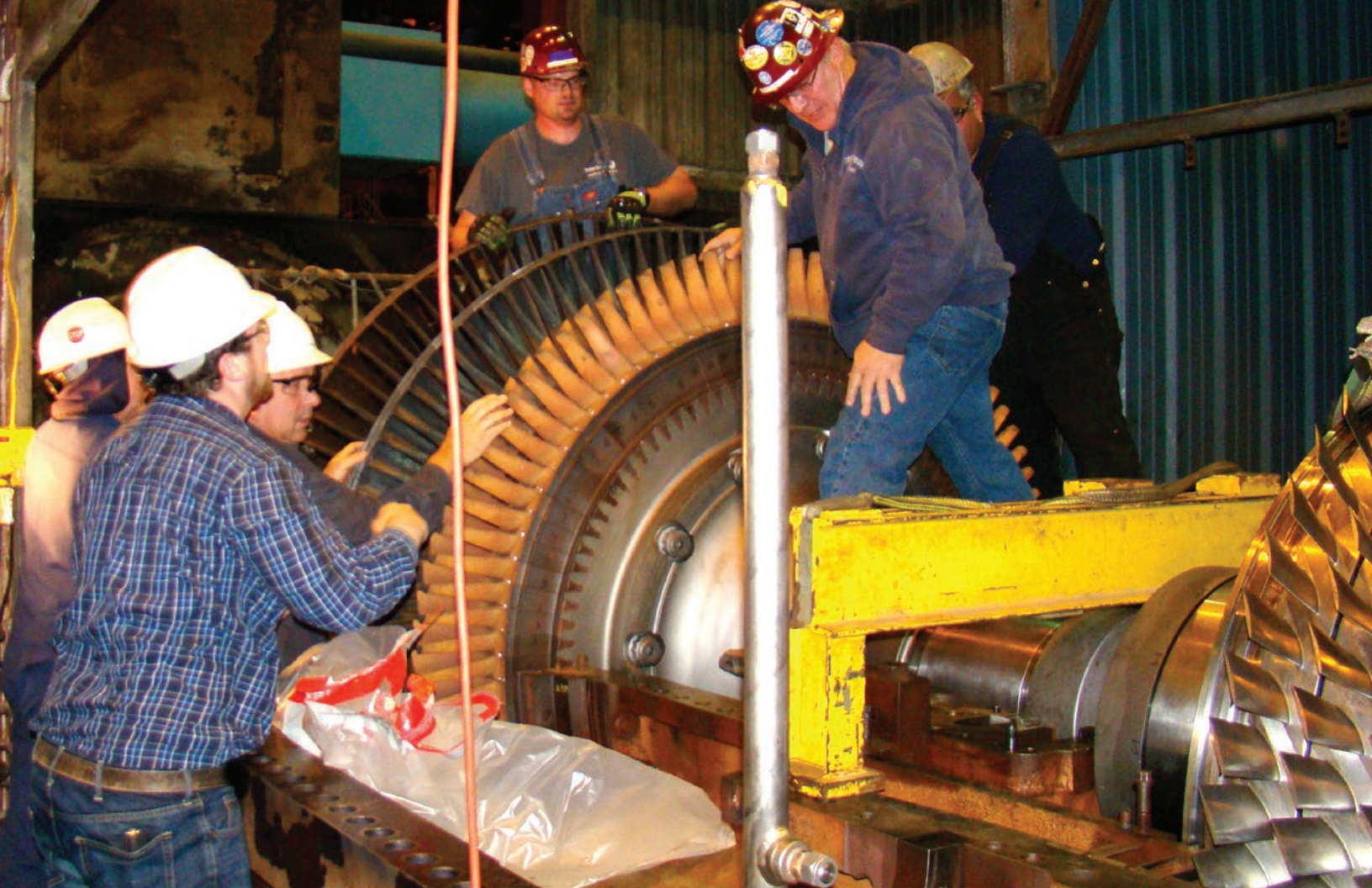
MMWEC staff and contractors align the turbine rotor in Intermediate Unit 1A as part of a life extension program for the Stony Brook power plant.
